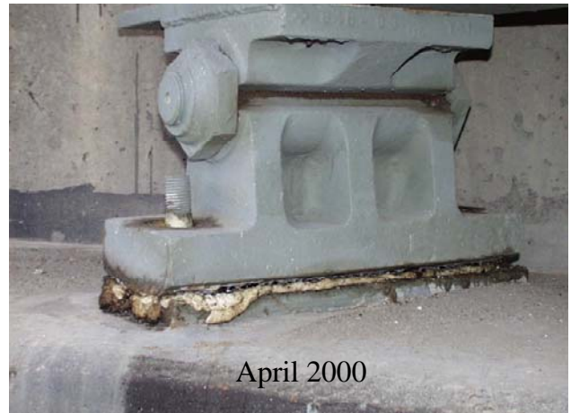
Figure 6 – Rocker Assembly Inspection – April 2000
