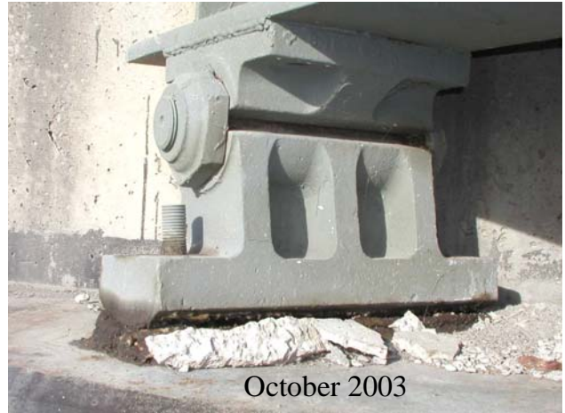
Figure 7 – Rocker Assembly Inspection – October 2003
