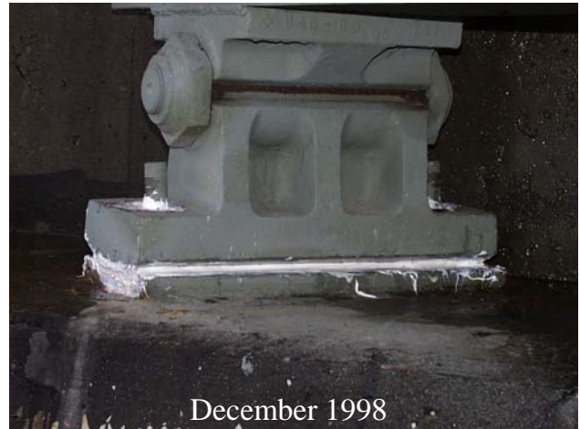
Figure 5 – Rocker Assembly After Gel Application - December 1998
