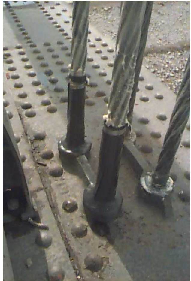
Figure 10 – Bridge Stay Finished Application – March 2004
