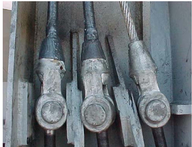
Figure 3 - US Navy Deck Edge Elevator Corrosion Remediation
